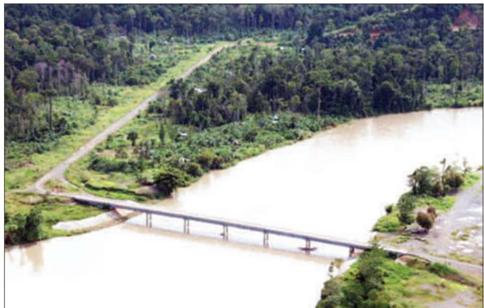
Ramu NiCo-MCC built the longest Ramu Bridge connecting Bundi LLG and Usino LLG today serves thousands of people. In the past, locals use dug-out canoes to cross the dangerous Ramu River
