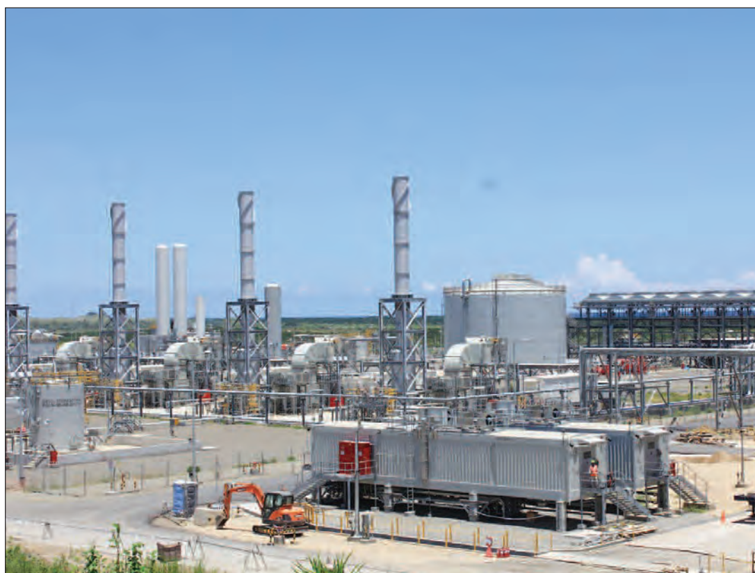
LNG Gas project site in Napanapa Central Province. Fail photo.
