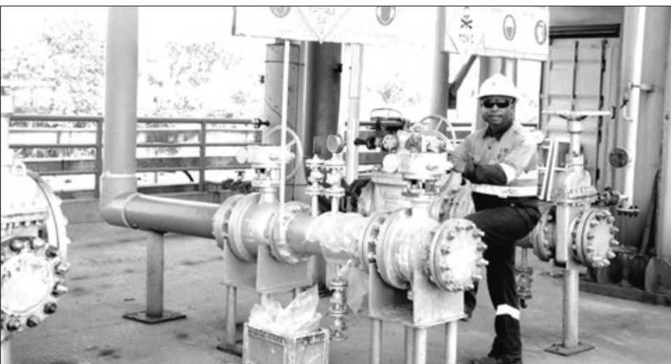
Tim lida long Basamuk Port, Saluk Wang i soim tupela valv bilong alkalain na hevi fiul long go long sip.
