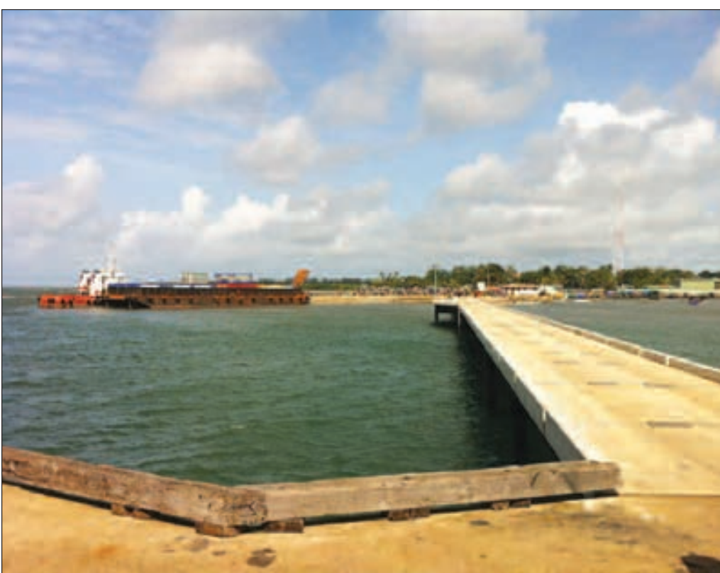
NUPELA BRIS BAI HELPIM DARU: Hia em nupela Trestle Bris bai helpim ol pipel na Daru i lukim sampela developmen. Poto: PNGSDP Midia
