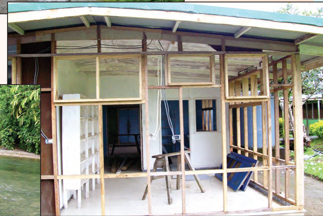
UNDER CONSTRUCTION: One of the buildings under construction at the research training centre, Konga, South Bougainville.
