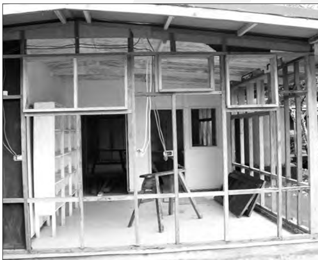
NEW STAFF HOUSES: One of the PNGSDP funded staff houses under construction at Tonu High school, Siwai.
