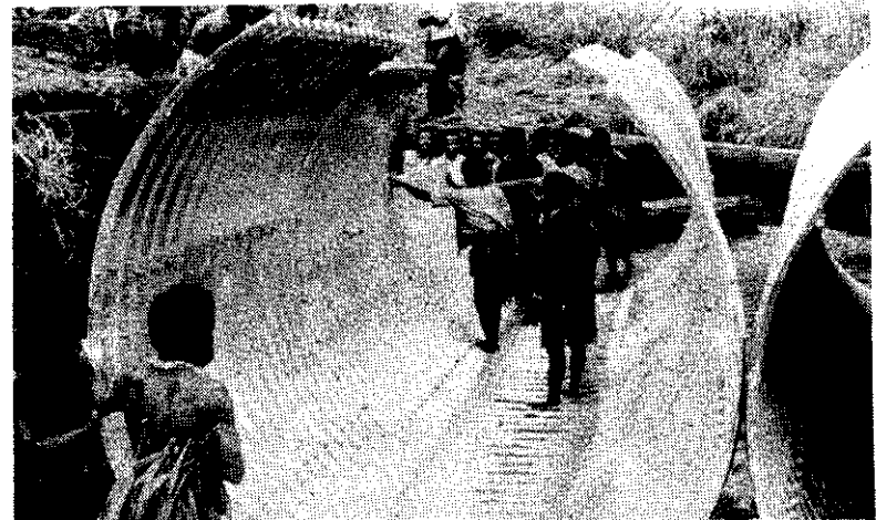
(4) Graham Campbell, em i wanpela ensinia, i wok hia wantaim ol pipel bilong Saten Hailans i wokim wanpela bikpela mambu bilong wara i brukim rot i stap namel long Ialibu na Tambul. Nau wara i stap aninit long rot na ol pmv i ken ran gut.
